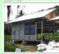
Building houses in Pulo Aceh
